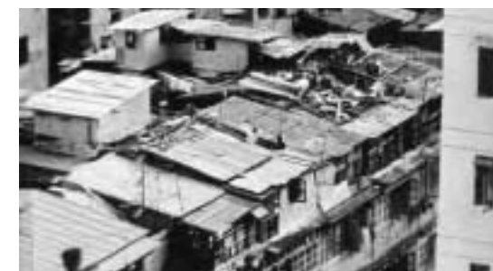
Roof-top squatters in Hong Kong, 1978.
