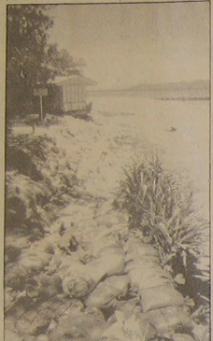
Visitors to Green Island in the Cairns Section, Great Barrier Reef Marine Park as greeted by the sight of thousands of sandbags, an attempt to protect an incorrectly sited resort from erosion.
