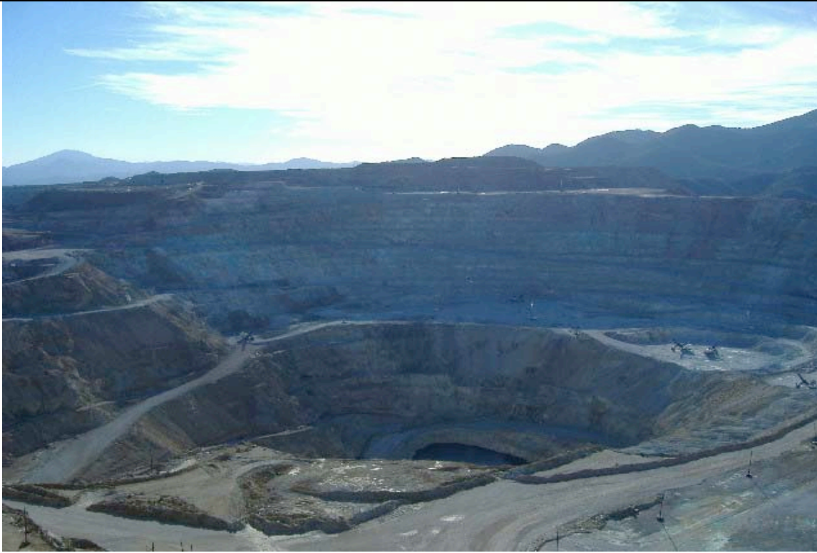
Photo No. 2: View of active excavation & blasting area of Mine Operations Department
