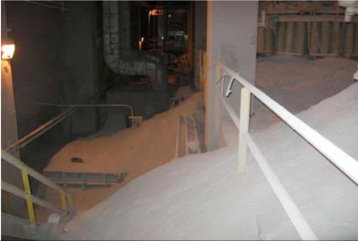
Photo No. 3: Working Conditions: Accumulated silica dust in Concentrator Building
