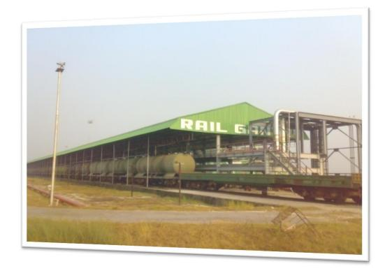
SMT has facilities for loading full BTPN Tank Wagon rake with product MS, HSD and SKO. It has facilities to unloading Tank Wagon HSD and SKO Tank Wagon rake.
