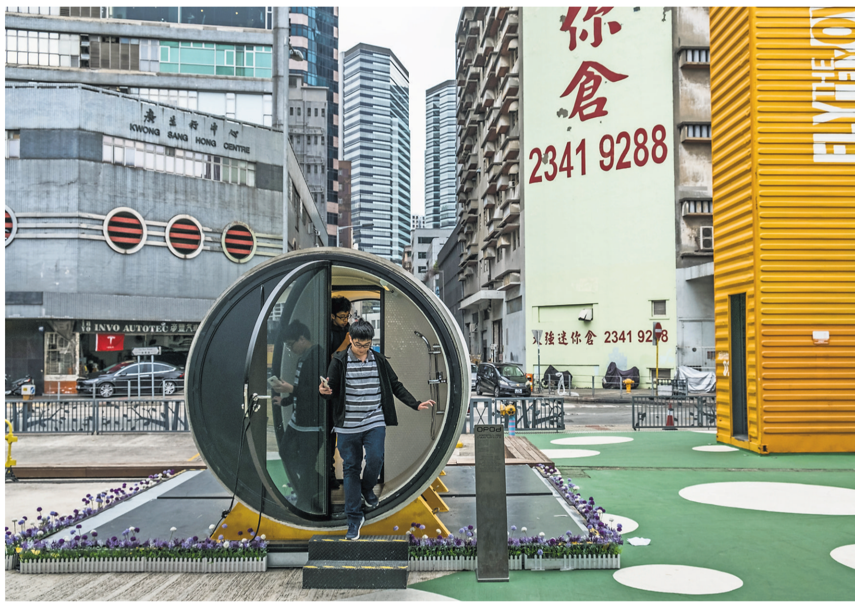
A prototype of the OPod in Hong Kong. Designed by the architect James Law, the OPod would create a living space of about 100 square feet out of concrete drainpipe.
