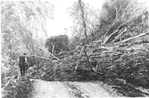
THIS LANDSLIDE AT LOT'S CREEK, Ky., was caused by strip-mining (photo by Mike Clark).
