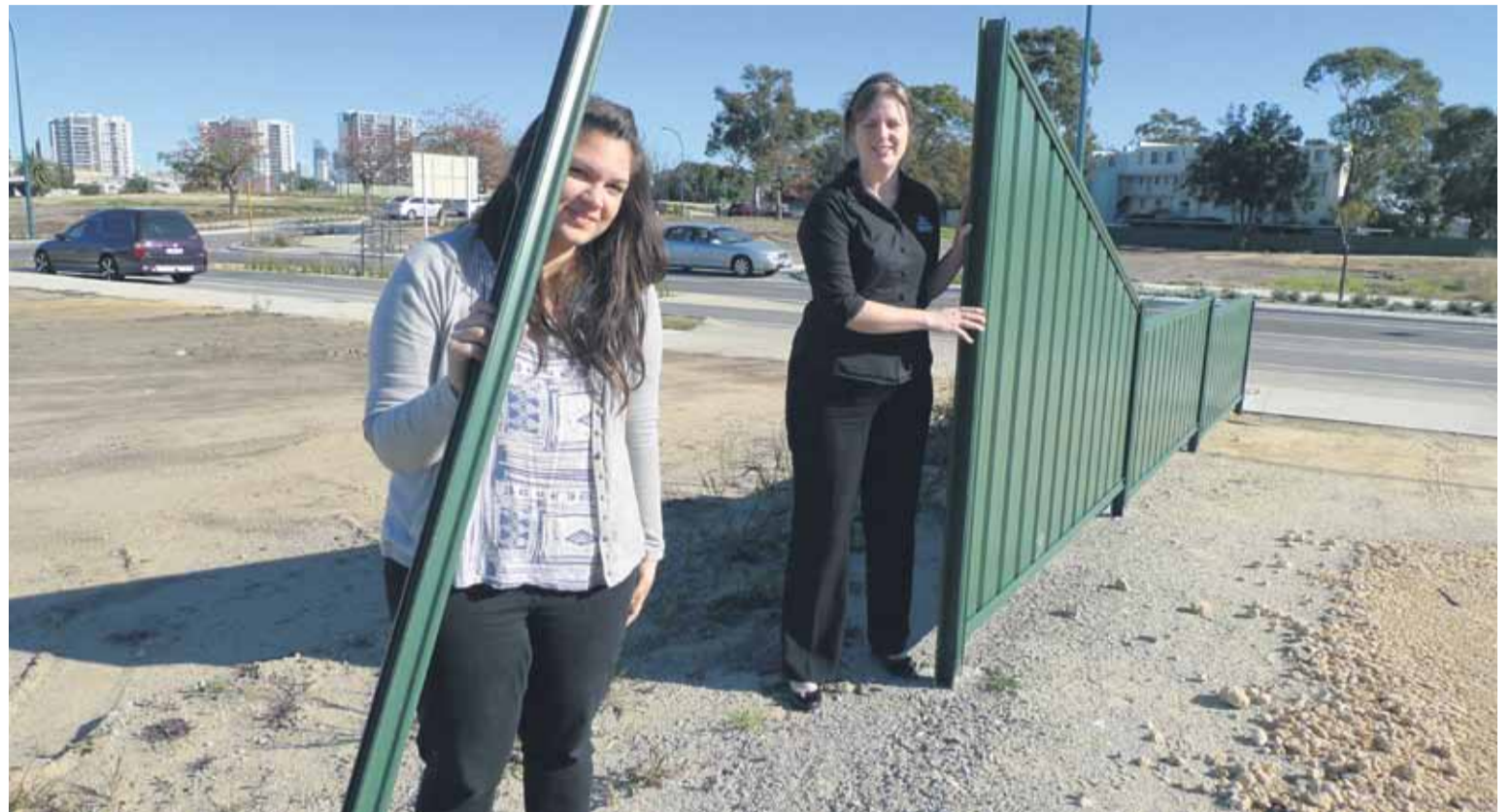
Bek D'Sylva (left) and Priscilla Penn from Baptist Churches Western Australia inspect some of the damage to the fences at the Baptist Ministry Centre in Rivervale following the destructive storms on 10 June.
