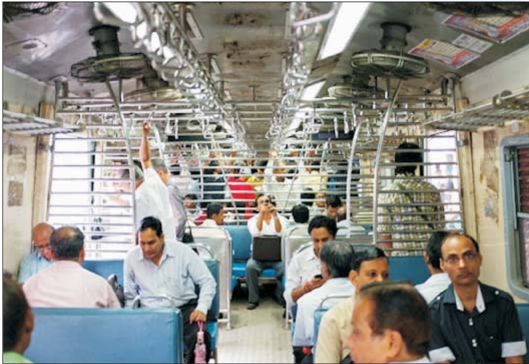
EMU fitted with LED lighting
