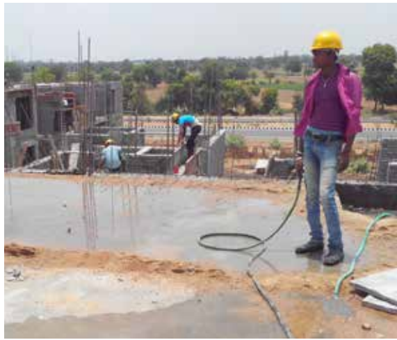
Curing of floor slab concrete
