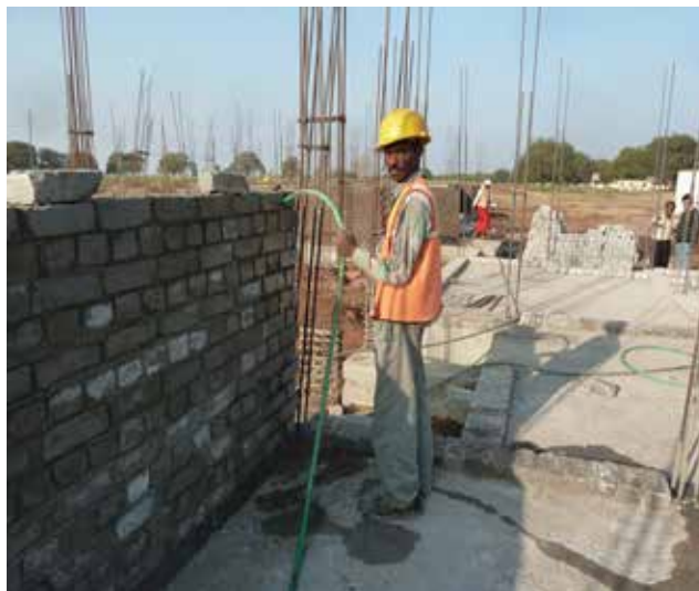
Figure 46. Curing of masonry walls.
