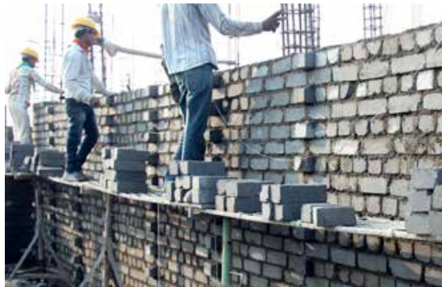
Wall construction at higher elevations
