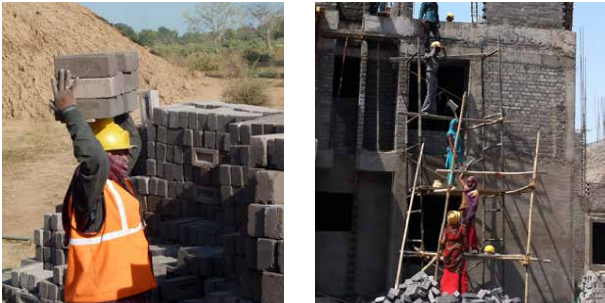
Figure 34. Transporting bricks at the construction site.
