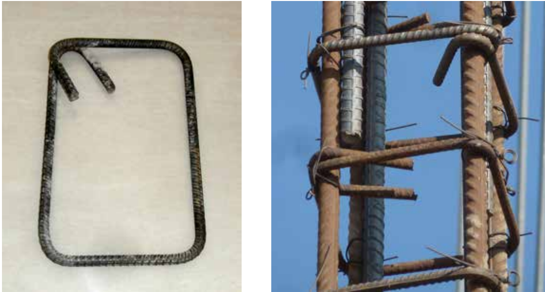
Figure 48. Transverse reinforcement (ties) for RC tie-columns - note 135 degree hooks.
