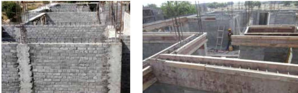
Reinforcement cages set in place
