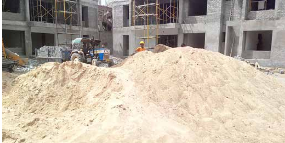
Figure 24. Sand supply at the construction site.
