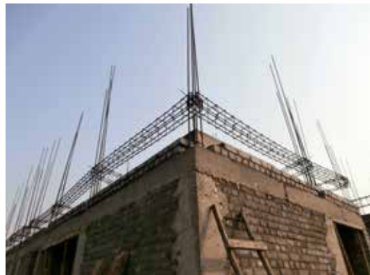
a) Tie-beam reinforcement set in place
