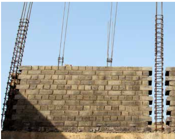
Figure 10. Masonry wall between adjacent tie-columns (construction in progress).
