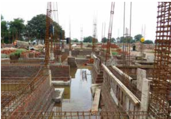
Plinth band reinforcement cage set in place
