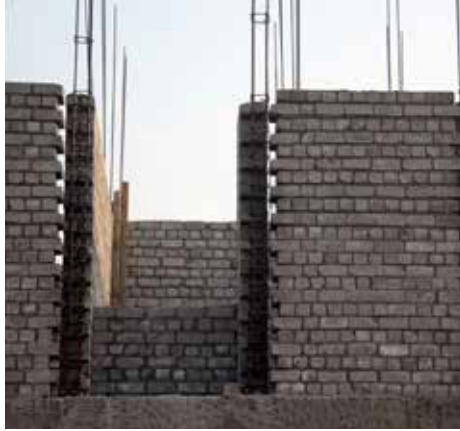
a) RC tie-columns before formwork was set in place
