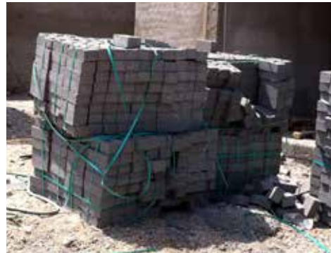
FALG bricks at the construction site
