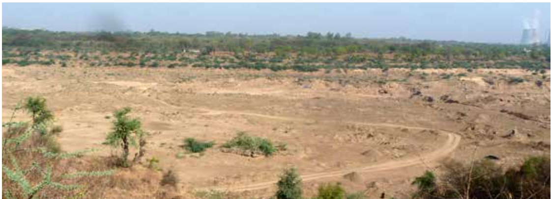
Figure 27. IITGN campus site before construction - note thermal power plant at the far right (April 2013).
