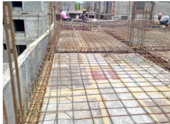
Figure 15. Tie-beam and slab reinforcement.
