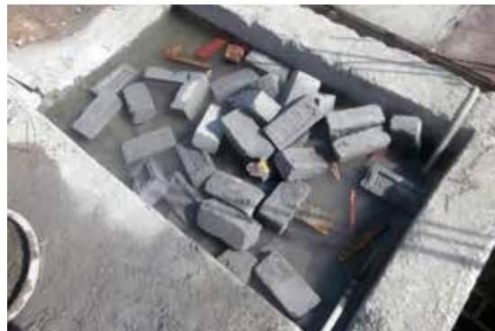
Figure 35. Bricks immersed in water before construction.
