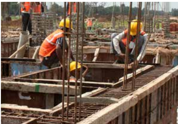
Tie-column longitudinal reinforcement anchored into plinth band
