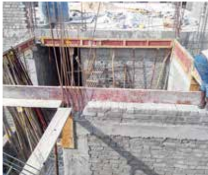
a) Setting in place interior formwork for tie-beams
