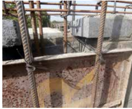
b) Steel wire ties were used to fix shuttering in place
