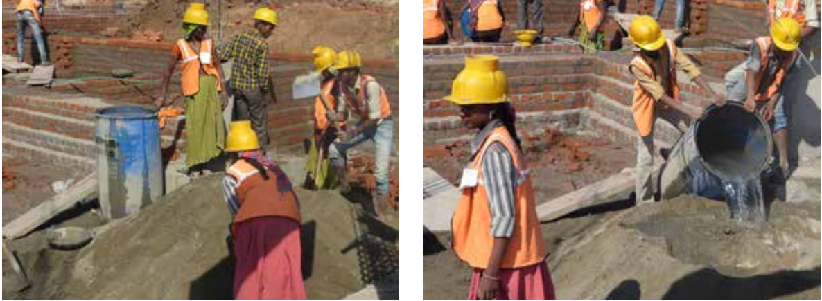
Figure 31. Construction at the plinth level - mortar preparation.
