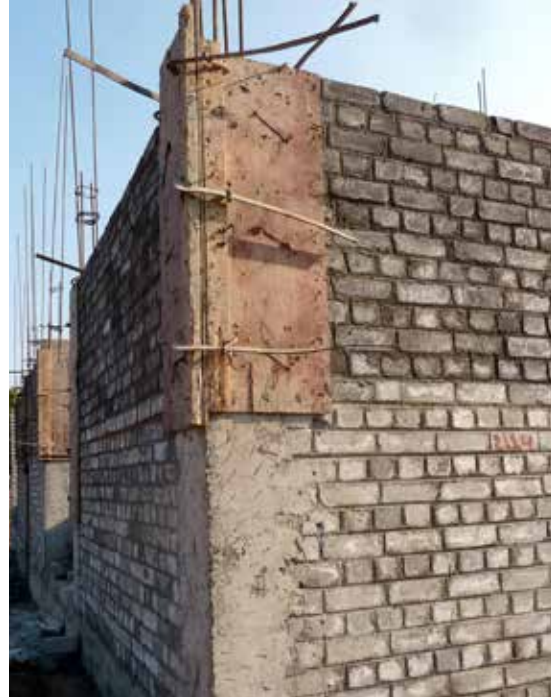
Figure 13. Formwork in place at upper portion of a RC tie-column.
