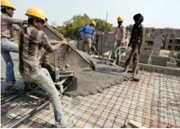
Pouring concrete for the floor slab
