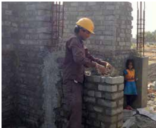
Mason laying a mortar bed joint
