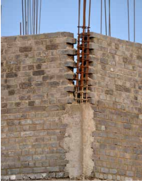
Figure 12. Concrete construction completed at lower portion of a RC tie-column.
