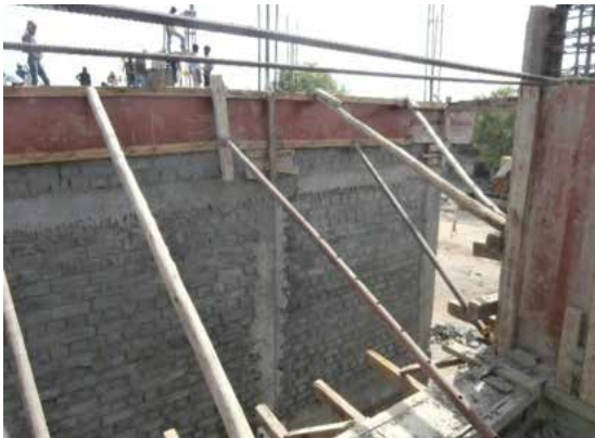
Figure 14. Formwork for tie-beams.
