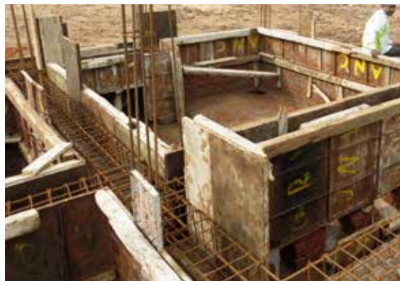
Formwork for plinth band construction
