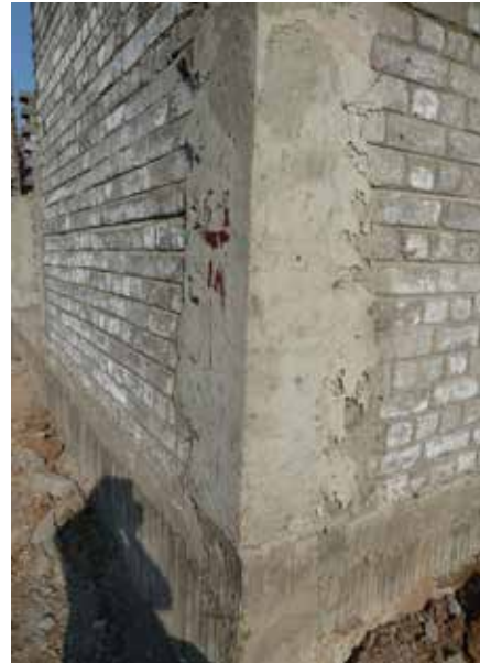
b) Exterior tie-column at a wall intersection
