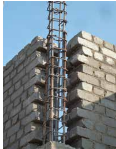
b) Tothed wall edges at a corner tie-column
