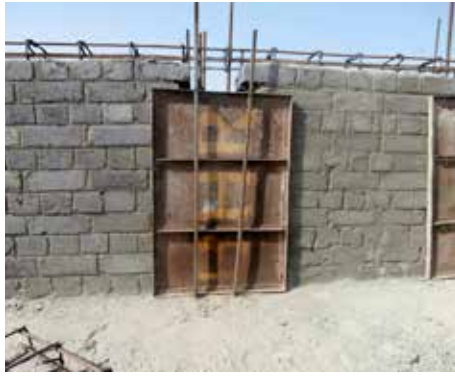
a) Shuttering in place at an interior tie-column
