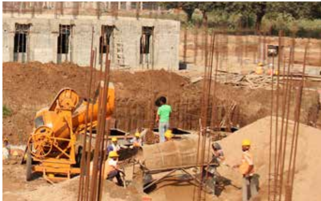
Figure 36. Mortar mixing at the construction site.
