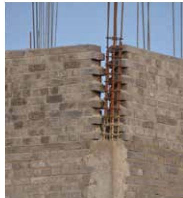
Tie-column construction completed up to 1.5 m height
