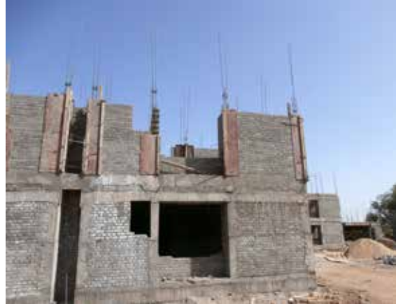
b) Formwork for RC tie-columns set in place
