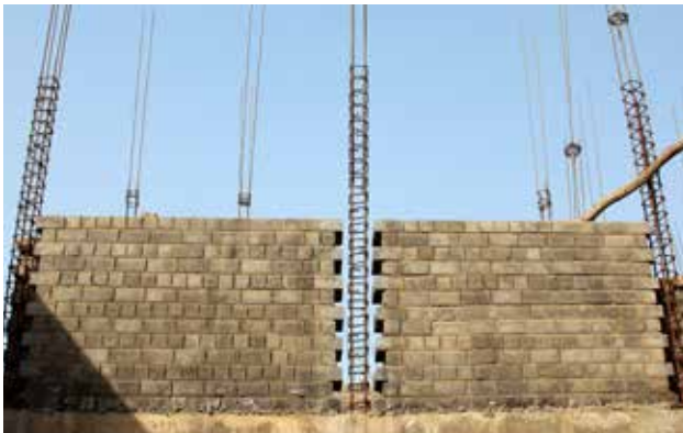
Wall construction completed up to 1.5 m height (one lift)
