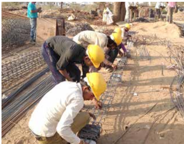
b) Steel reinforcement cages assembled at the site
