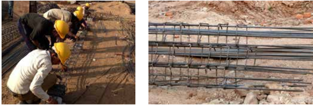
Figure 43. Construction workers assembling reinforcement cages for RC lintel bands.
