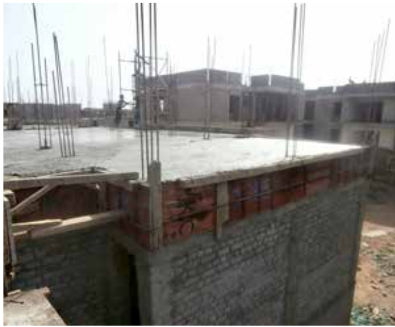
Completed floor slab construction
