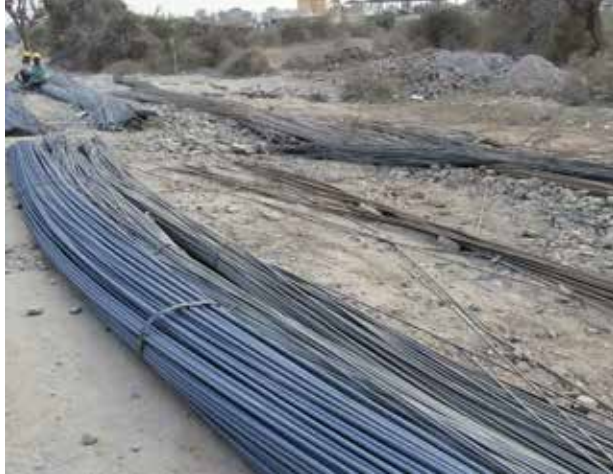
a) Steel delivered at the construction site
