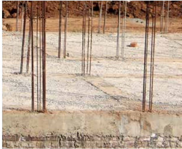
Figure 9. Tie-column longitudinal reinforcement at the plinth level.
