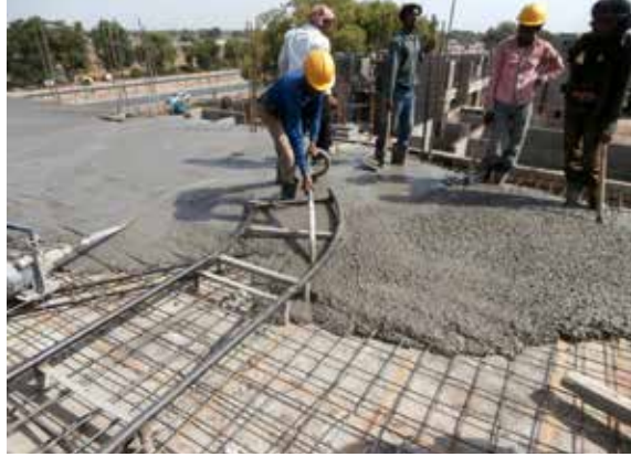
Concrete compaction with a needle vibrator
