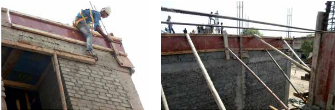
a) Setting in place exterior tie-beam formwork
