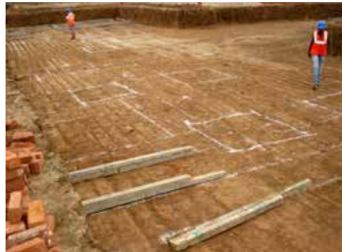
Figure 29. Construction workers marking foundation plan dimensions at the cleared ground.
