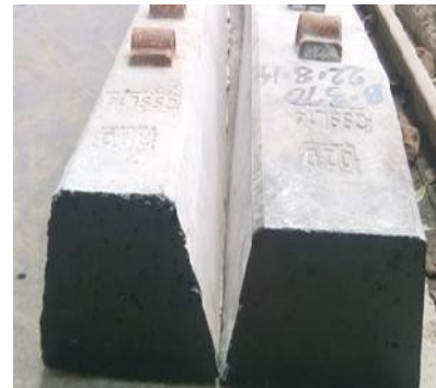
Existing 25t & wider sleeper
