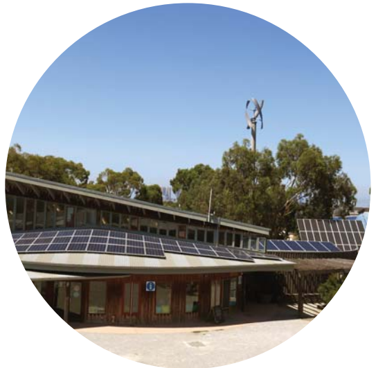
[above] New solar array on the Visitor Centre.
