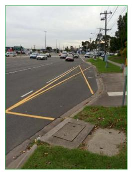
Figure 12 New line marking at bus stop to avoid confusion
