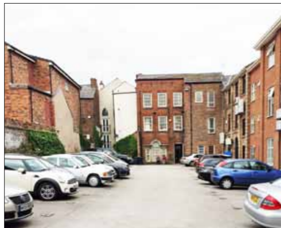
Rear elevation from the car park
