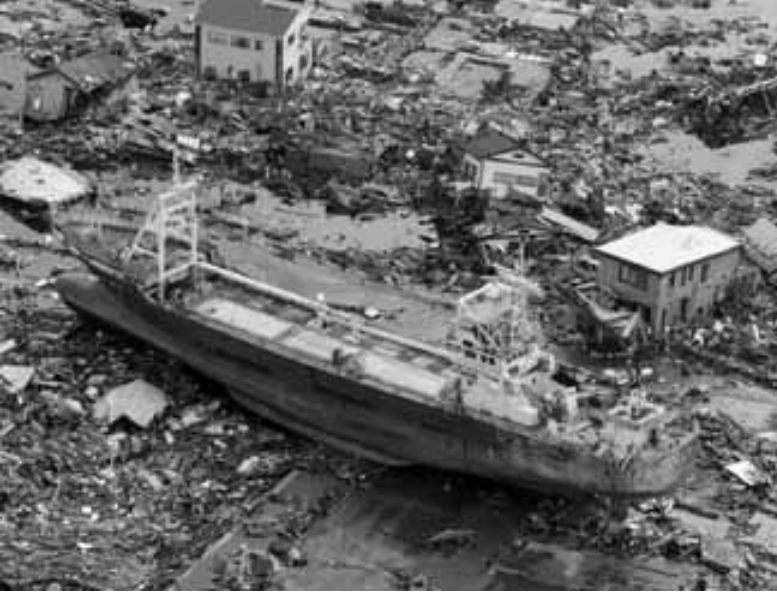
Damage from the March 11 tsunami.
