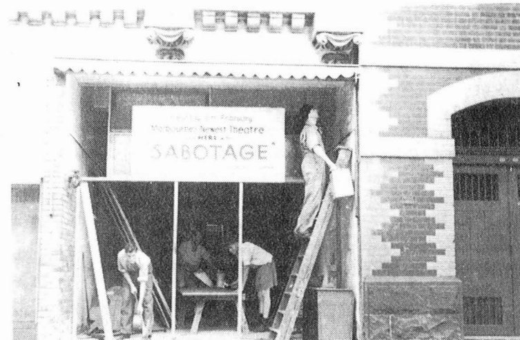
Above and left, members building Flinders Street Theatre
