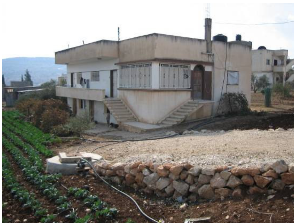
A rainwater harvesting scheme with pipe extending from the roof to a cistern, Jalboun
