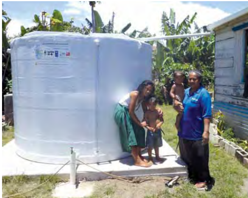
A pumphouse (top) and one of the 10,000 litre water tanks (bottom).
