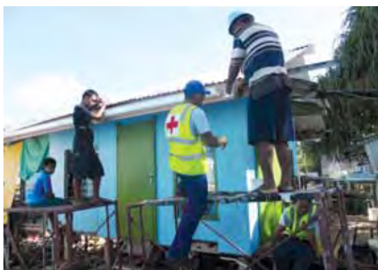
Repairing water infrastructure on Tuvalu.
