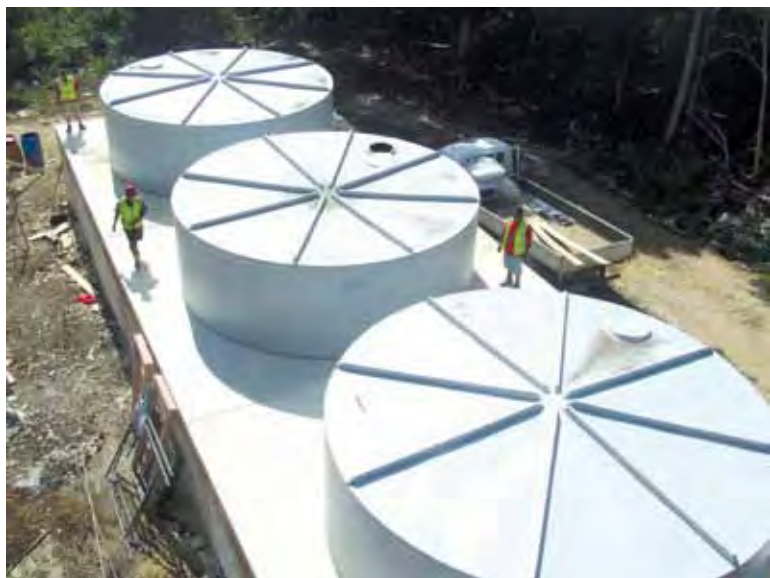
The three 45,000 litre tanks installed.
