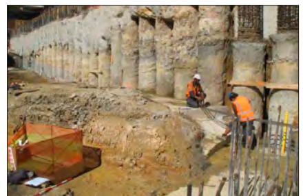
WG building site where well was discovered.
