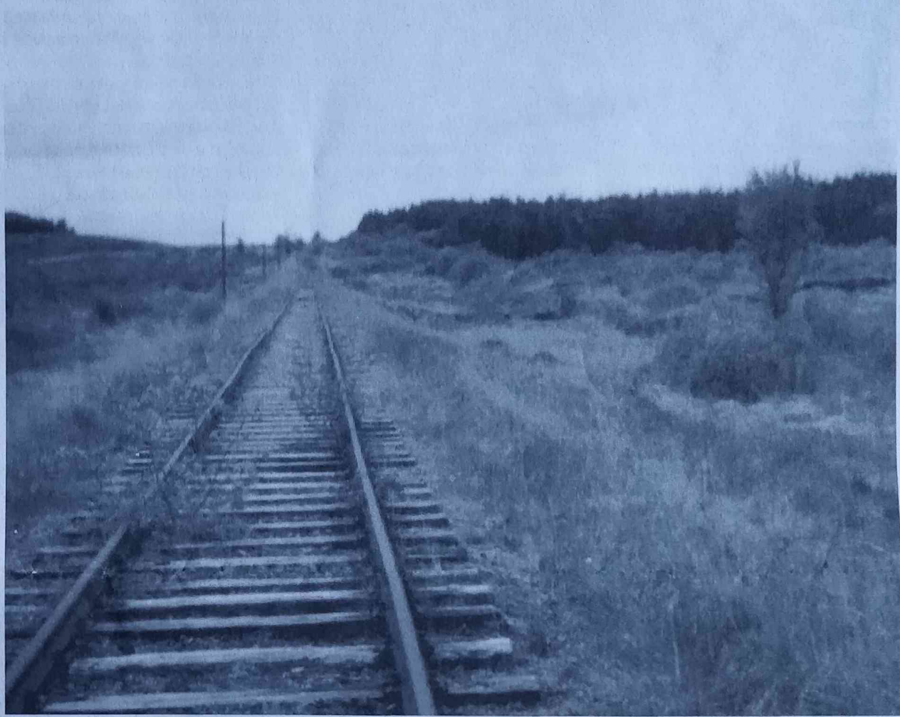
A vision of the future - an abandoned railway line
