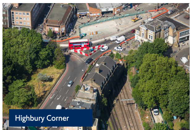
Structure and tunnel works
