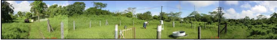
Figure 4. 180-degree view of the Afiamalu climate station enclosure. The building at the left (south) of the station houses the seismic monitoring and data transmission controls.
