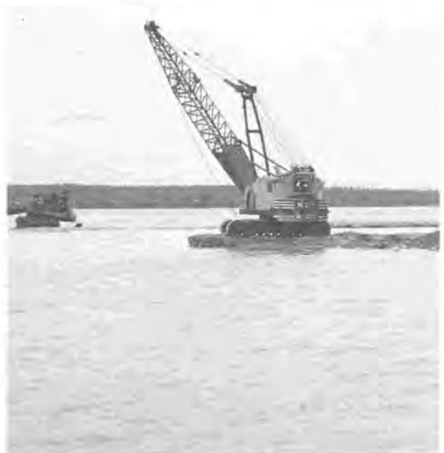
Coral fill material is dredged from the lagoon near Apia. (photo: Jennie Cary, reproduced courtesy of DLSE)
