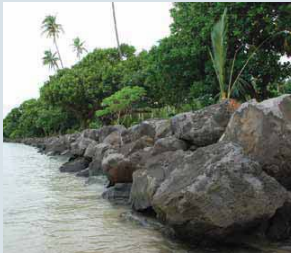
Shoring up the sea front (Vaitapu)
