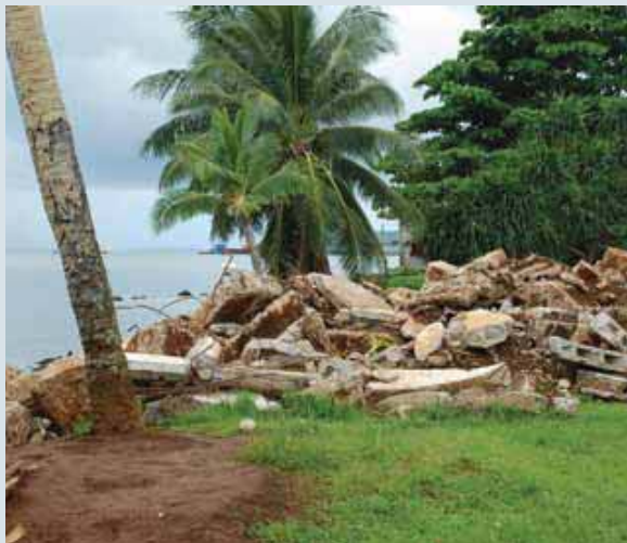
Shoring using building debris (Liku)
