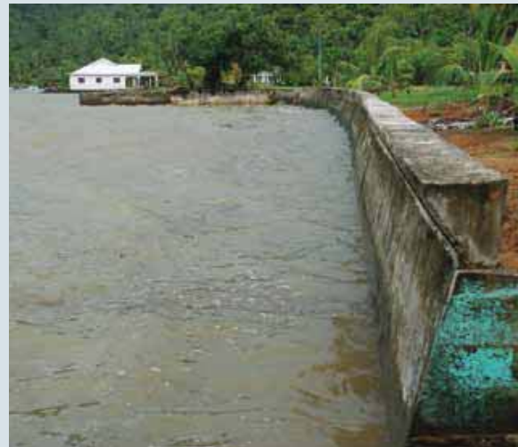
Protection wall (Gahi Bay)
