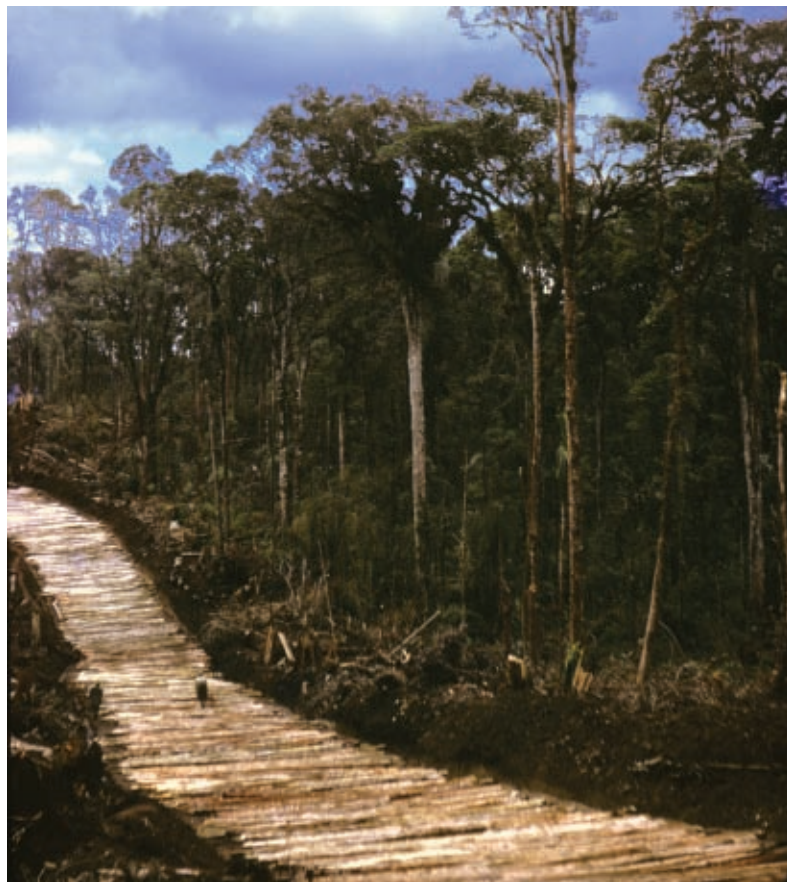
Plate 5: Logging in Nothofagus forests on Mt Giluwe. Note the extensive utilisation of felled trees in the 'cording' of the roads due to very muddy terrain. A person is visible in the middle of the road.
