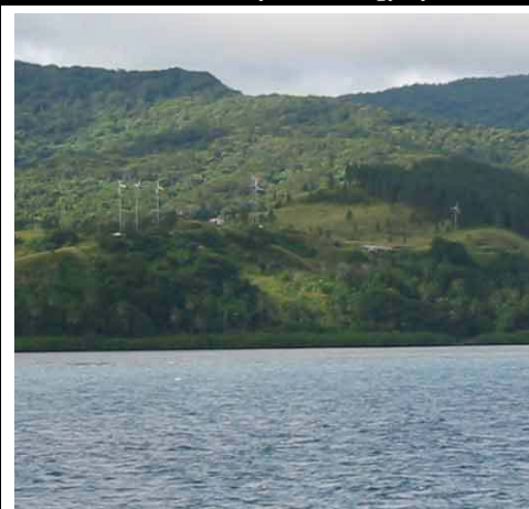
Figure 5-23 – The Nabouwalu Hybrid Energy System
