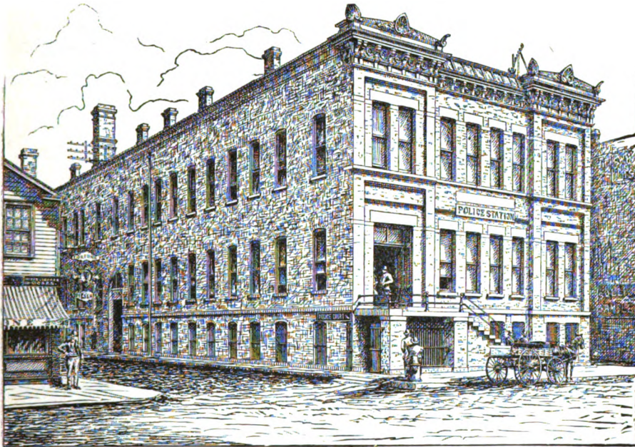
THE DESPLAINES STREET STATION.
