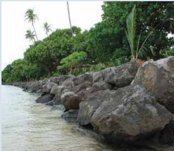
Shoring up the sea front (Vaitapu)
