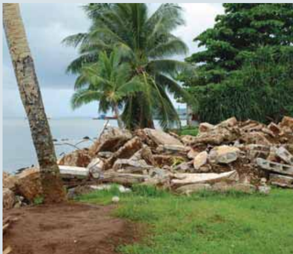
Shoring using building debris (Liku)
