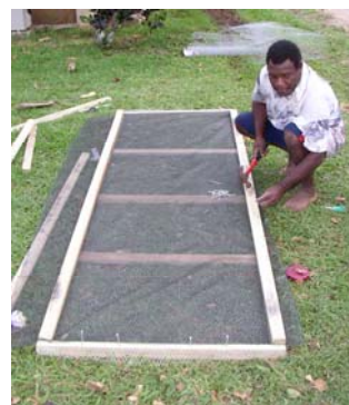
2. Stretching the chicken wire on the frame
