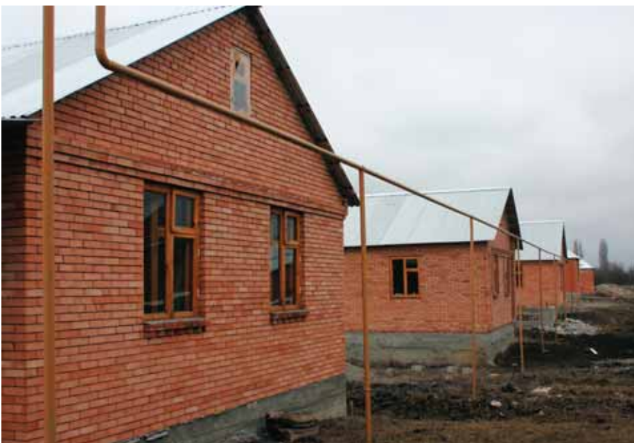
New houses constructed under the UNHCR and Swiss Agency for Development shelter programme. Ardonsky District, Republic of North Ossetia-Alania
