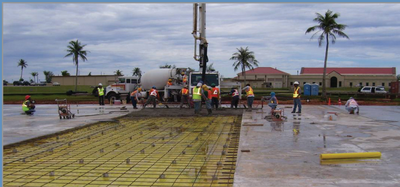
Contractors pour concrete for the foundation of a new 165,000 square foot base exchange building. Credit: U.S. Air Force photo
