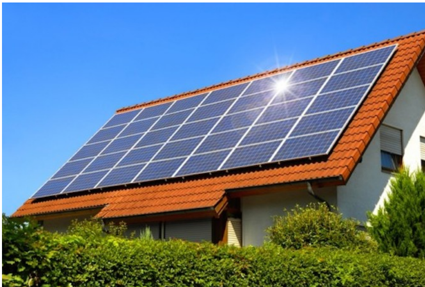
Figure 2.1: A rooftop array of photovoltaic cells.
