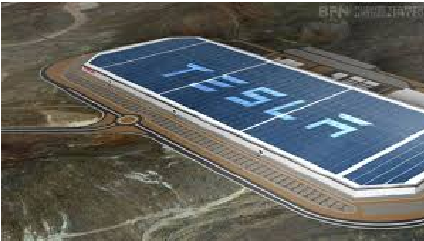
Figure 2.20: Tesla's Gigafactory 1 in Nevada produces improved lithium ion batteries. Energy for the factory is supplied by solar panels on the roof.
