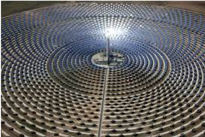
Figure 2.2: A solar thermal power plant. Arrays of heliostatic reflectors concentrate the sun's rays onto molten salt in the tower. The plant produces electricity at night because the salt remains hot..
