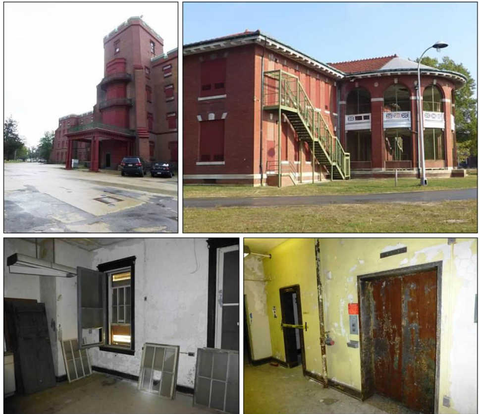
Figure 10: Images of Vacant Buildings on the St. Elizabeths Campus
