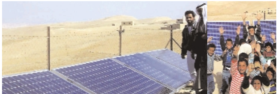
A new day for students in the remote village of Al-Kaabneh, on the West Bank, in Palestine. With photovoltaic solar panels, their school has electricity for the first time ever.
