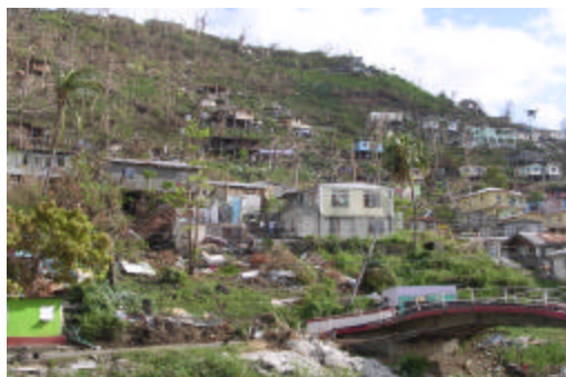
Photo 1 Damaged Housing in St. Georges
