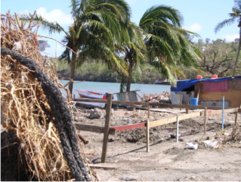
Photo 11 Reconstruction of housing at Soubise/Marquis
