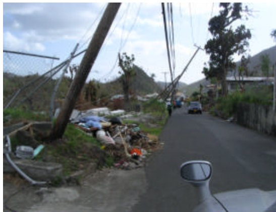
Photo 4 Typical Damage to Electric Poles
