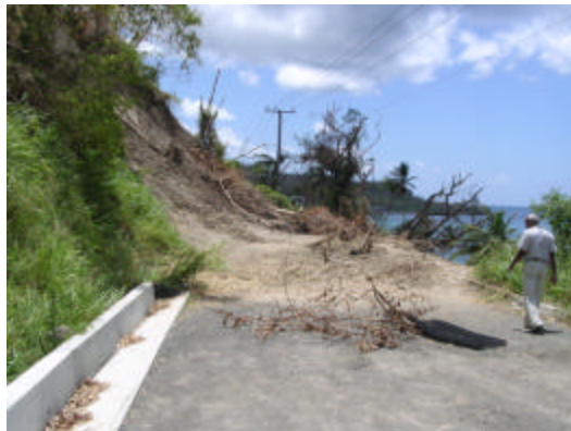
Photo 8 Land Slippage at Gouyave Blocking Western Main Road
