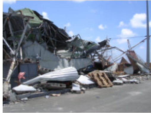
Photo 14 Damaged Geest Warehouse
