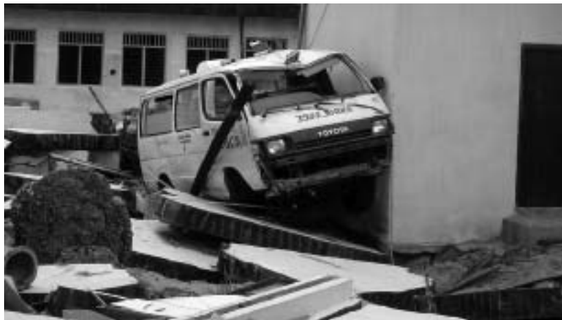
An ambulance crashed into a hospital from the force of the tsunami.
