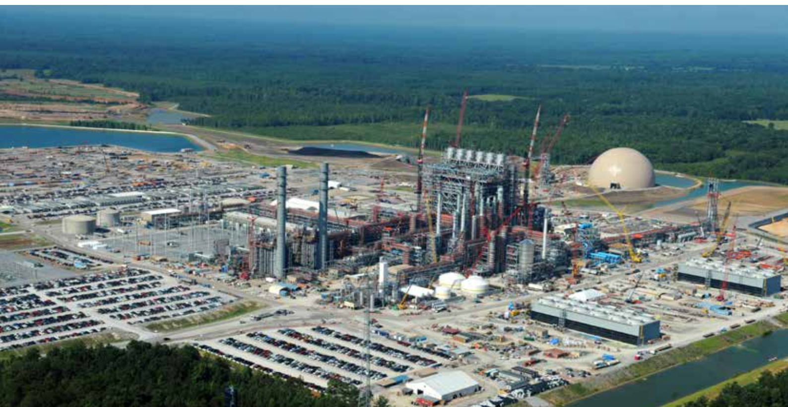
Building continues at the Kemper County Coal Gasification Plant, Mississippi, US
