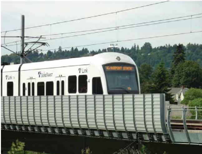
Existing sound wall along a portion of an elevated guideway.
