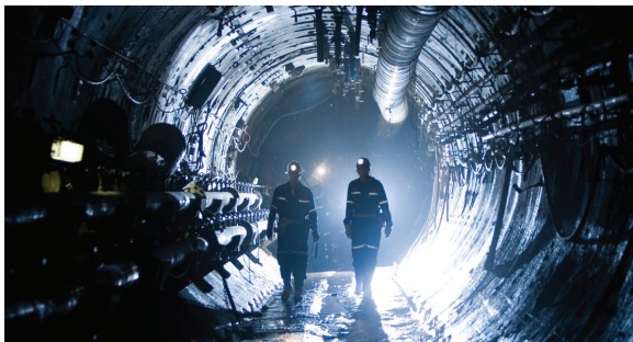
UNDERGROUND TUNNEL AT CIGAR LAKE MINE
