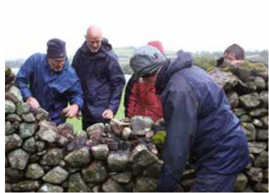
FIGURE 4.6 Volunteers repairing a stone wall
