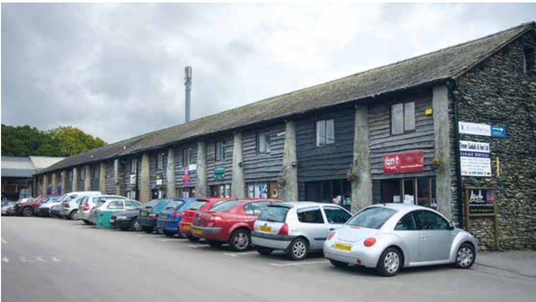
FIGURE 4.9 The re-use of Staveley Mill Yard. It now provides a number of employment and retail units.
