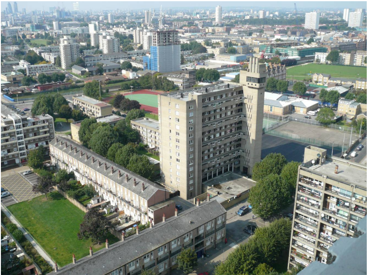
Figure 1: View across the Brownfield estate in Poplar, east London from the Balfon Tower, built during the mid 1960s and designed by the Hungarian born architect Ernő Goldfinger. The estate has a range of medium and high density housing, including the Balfon Tower itself, which stands 84 metres and 27 stories high and contains 146 flats. Photograph taken in 2008 by Rodney Harrison.
