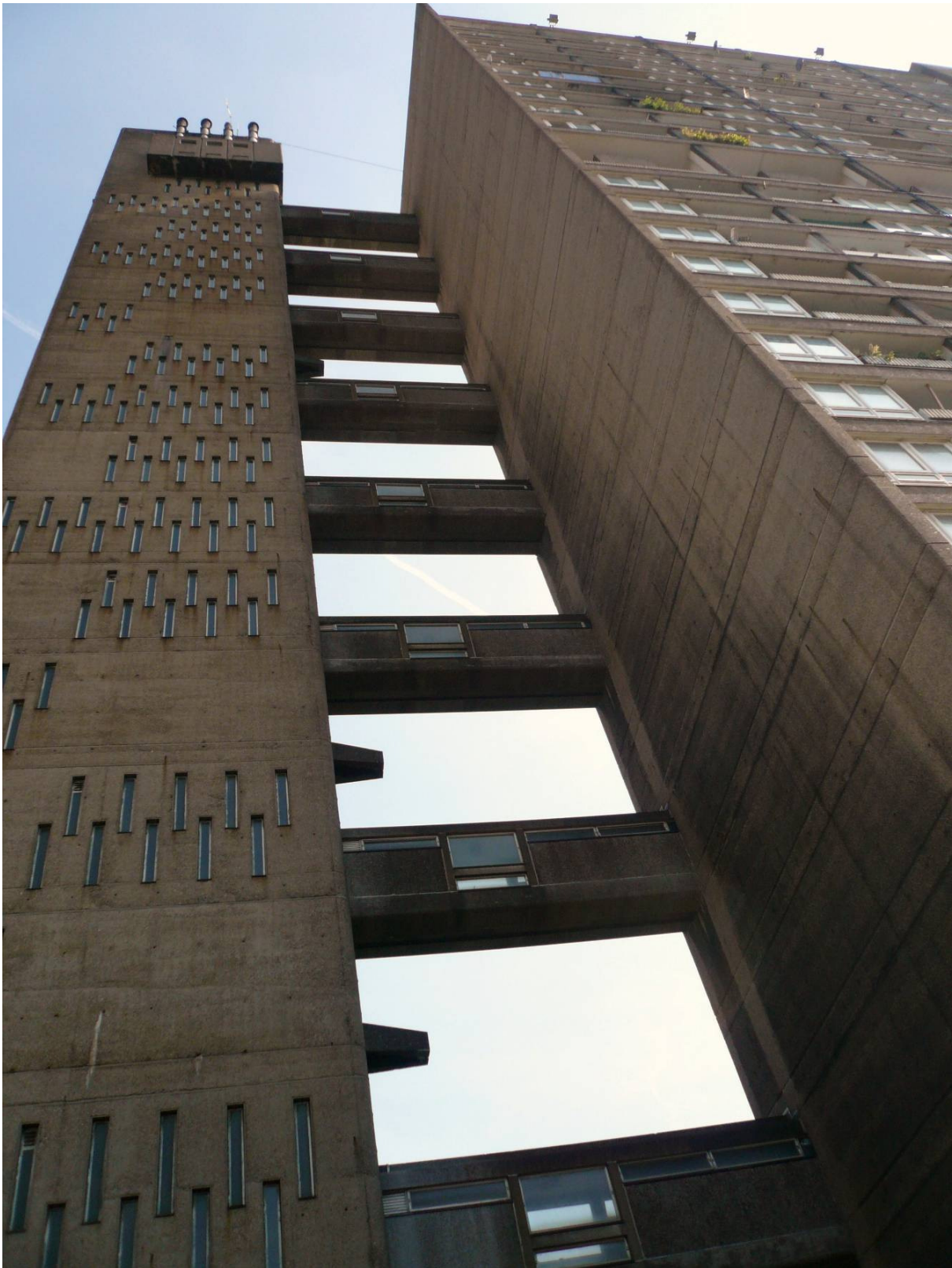
Figure 2: View of the Balfron Tower showing separate lift and services tower connected by walkways to the main block. Photograph taken in 2008 by Rodney Harrison.
