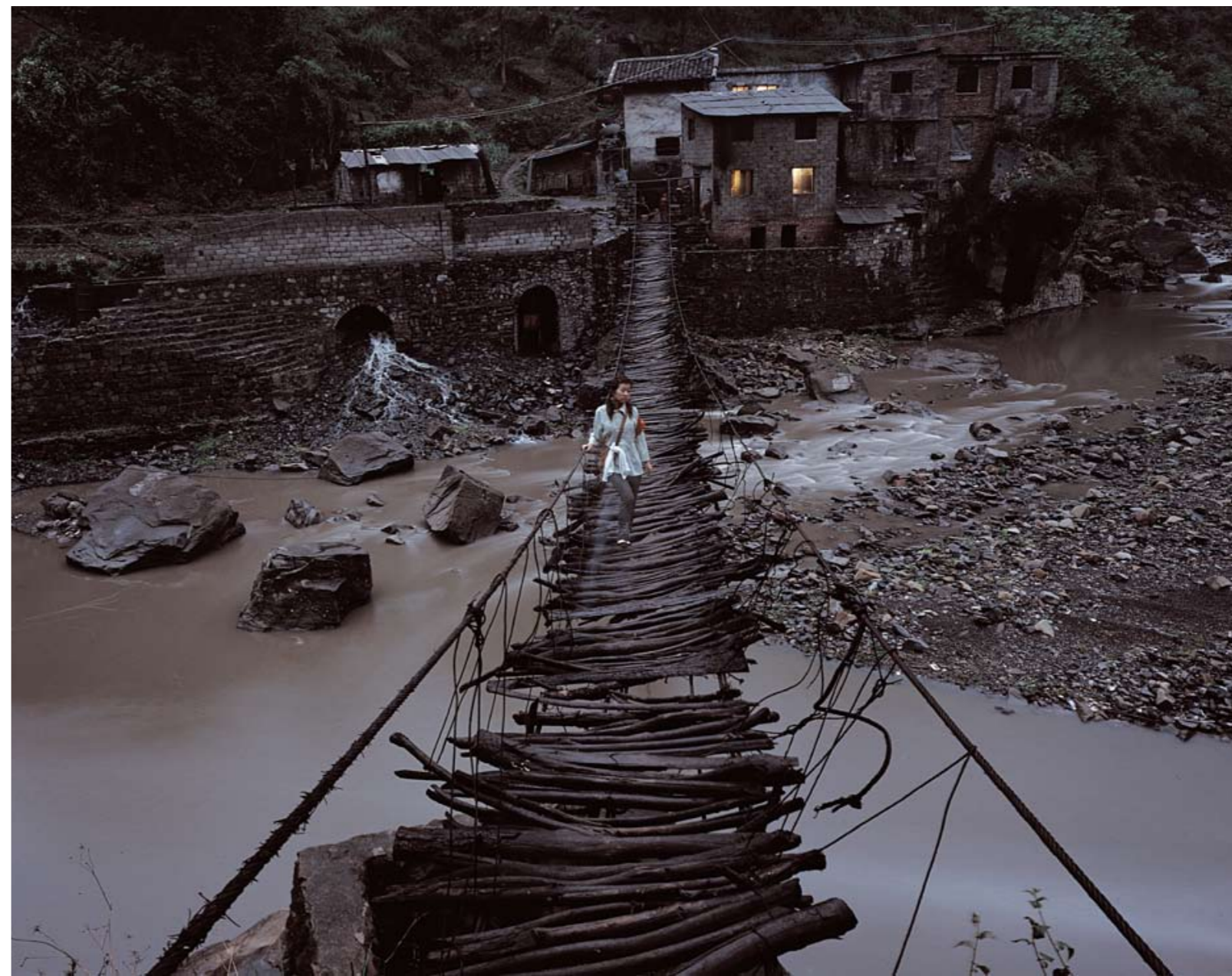
THIRD FRONT — CABLE BRIDGE 2005
