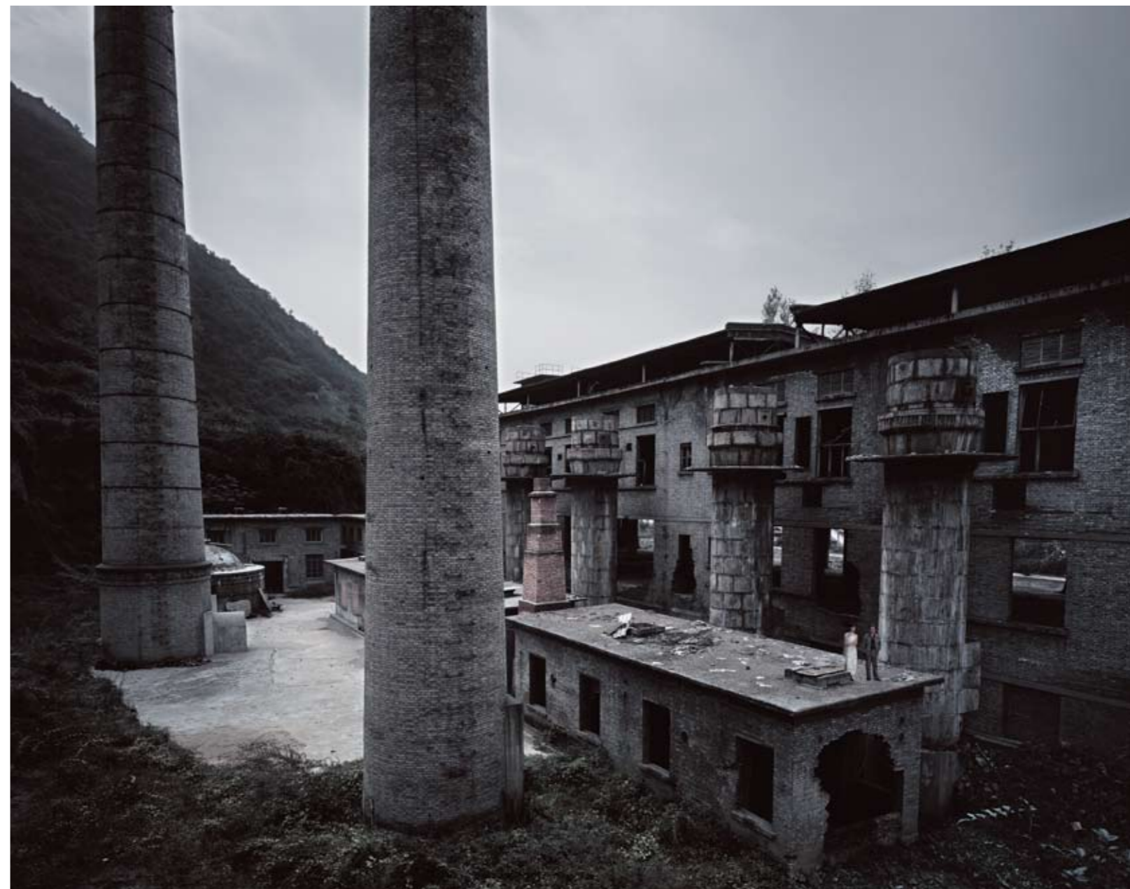
THIRD FRONT — FENGYANG COKE PLANT 2006
