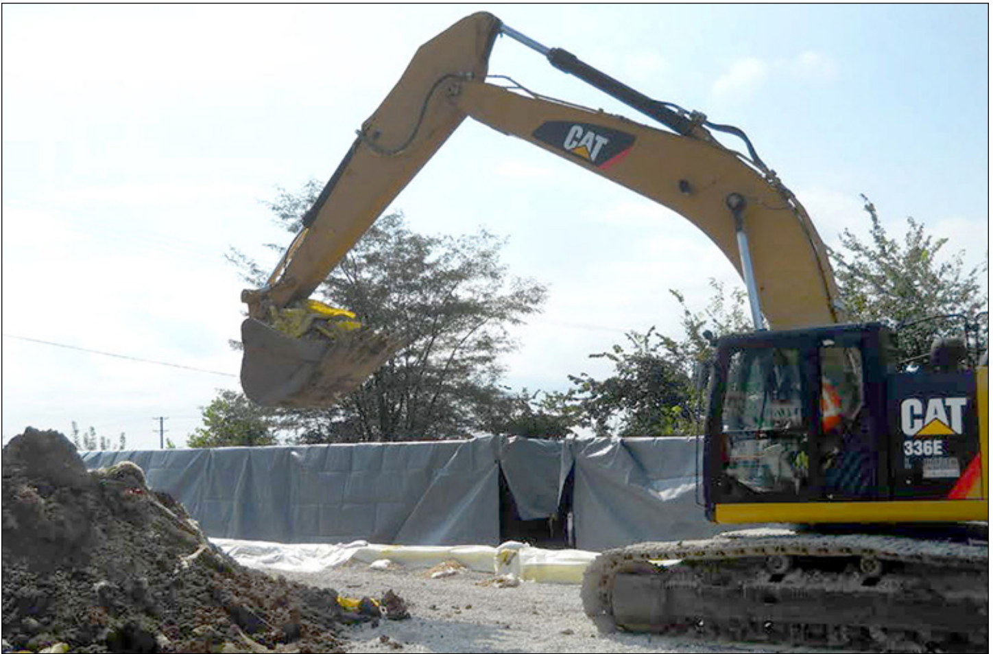
During the first shipping campaign at the Iowa Army Ammunition Plant, approximately 1,900 cubic yards of depleted uranium-contaminated soil were loaded onto railcars and shipped out of the installation.
