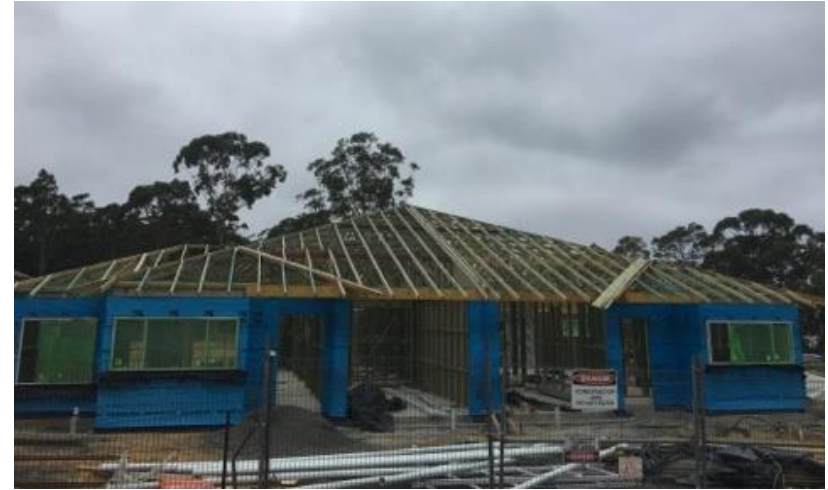
Island Point construction site
