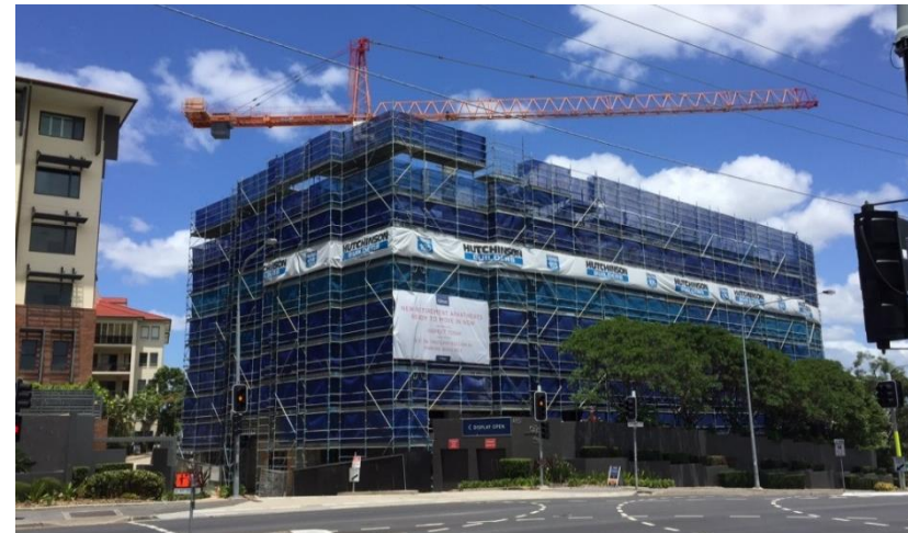
Clayfield construction site
