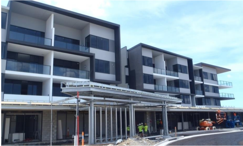
Springfield construction site
