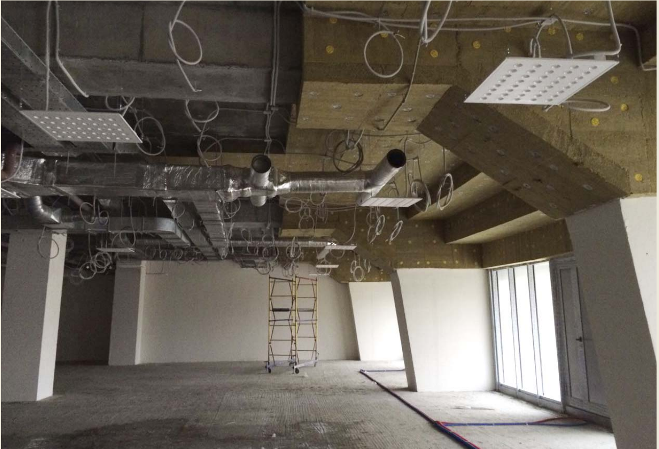
Installation of internal thermal insulation for walls and LED-based lighting fixtures
