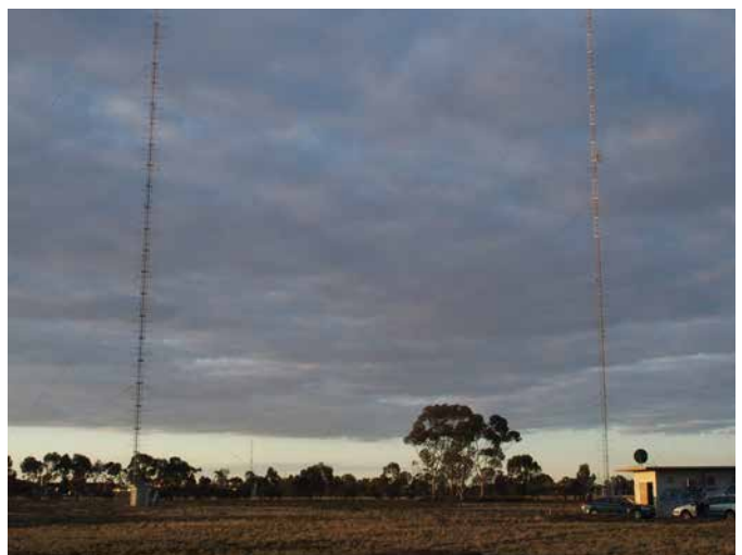
3CR transmitter site, Werribee
