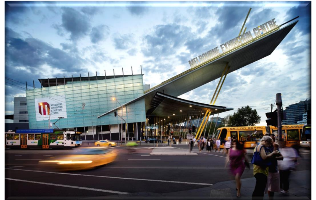
Investment in key infrastructure
