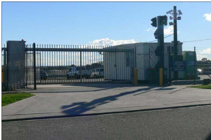
Example of an access control gate at a critical infrastructure facility.
