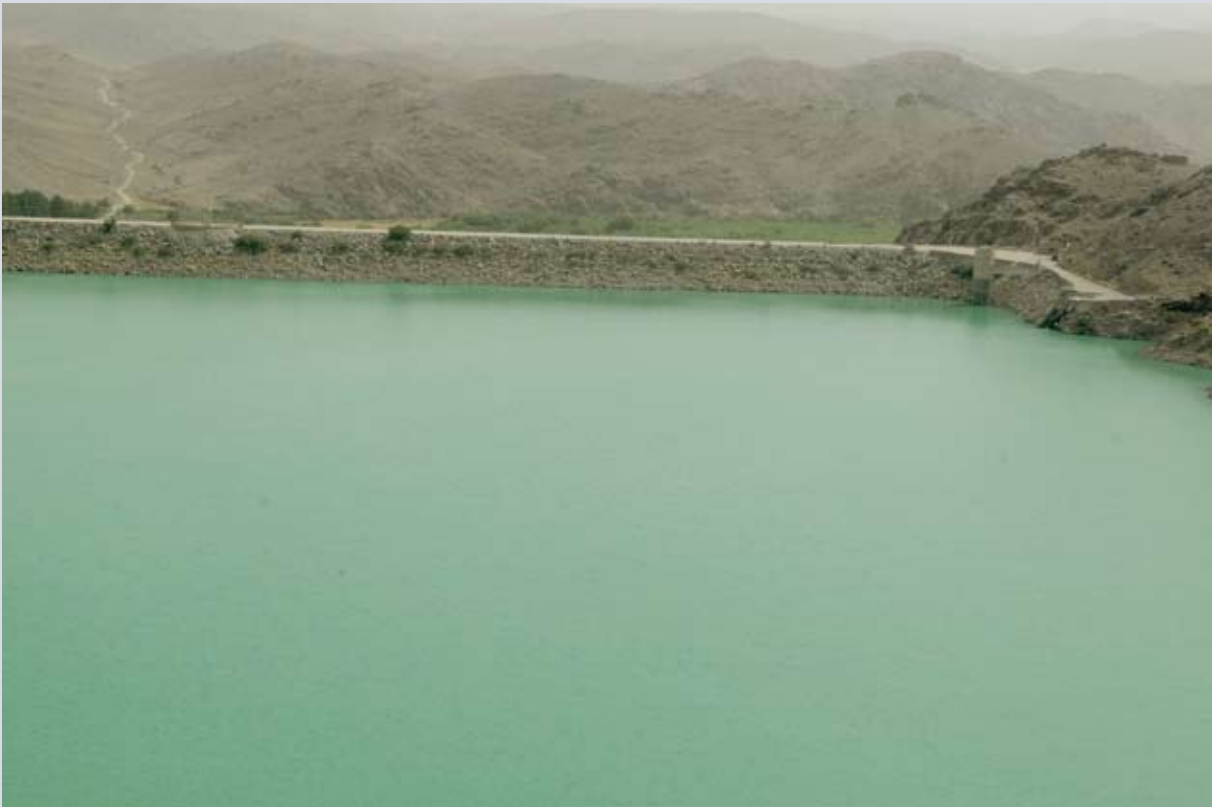
Aerial view of a portion of the Dahla dam in the Arghandab District, northern Kandahar, on 11 July 2008. (© Canadian MoD)
