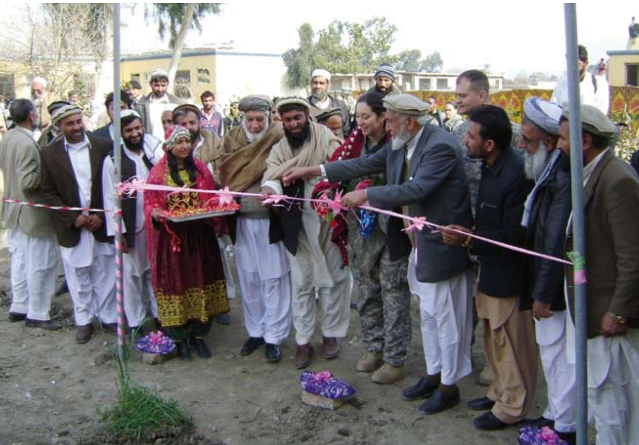
Provincial government representatives, local elders, school officials and PRT staff participate in a ceremony to mark the start of construction of a school for girls in the Behsood District of Nangarhar Province on 11 January 2009.
