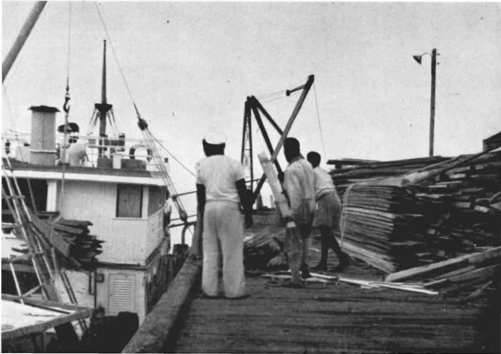
M.V. "Melbidir"—Loading Timbers, Red Island Point.
