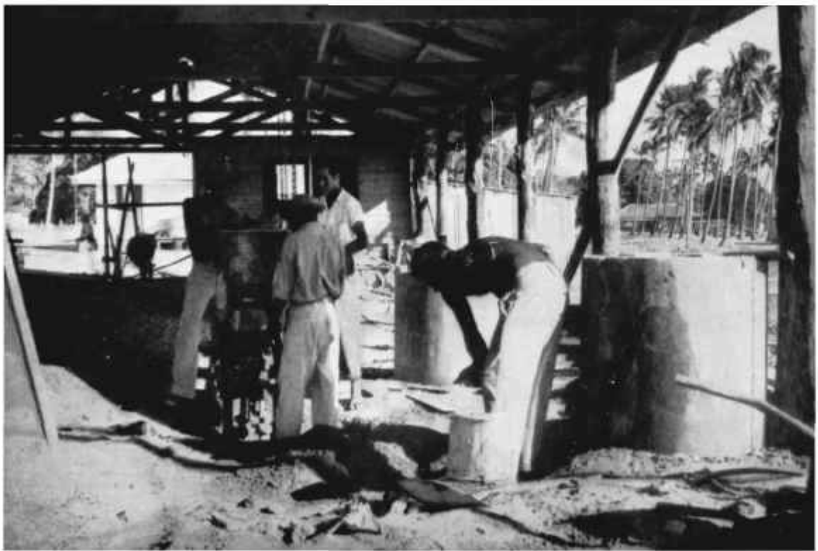
Cement Brick and Cylinder Making—Palm Island.
