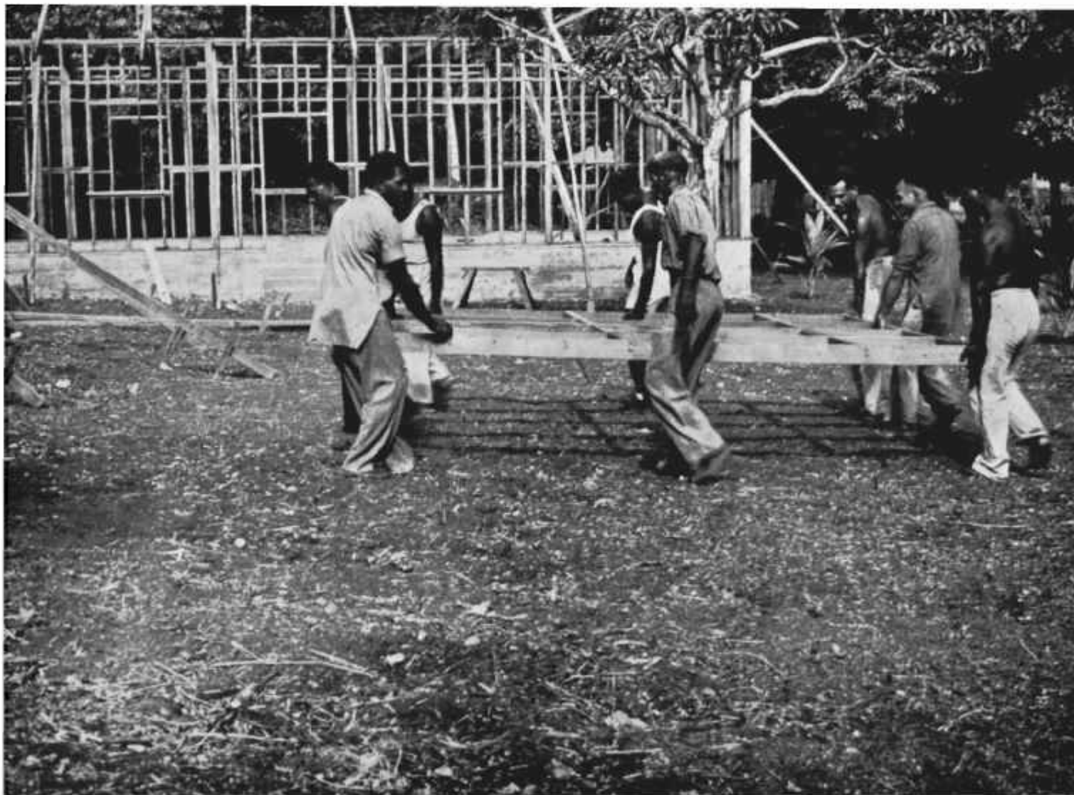
New School, Murray Island—in course of erection.
