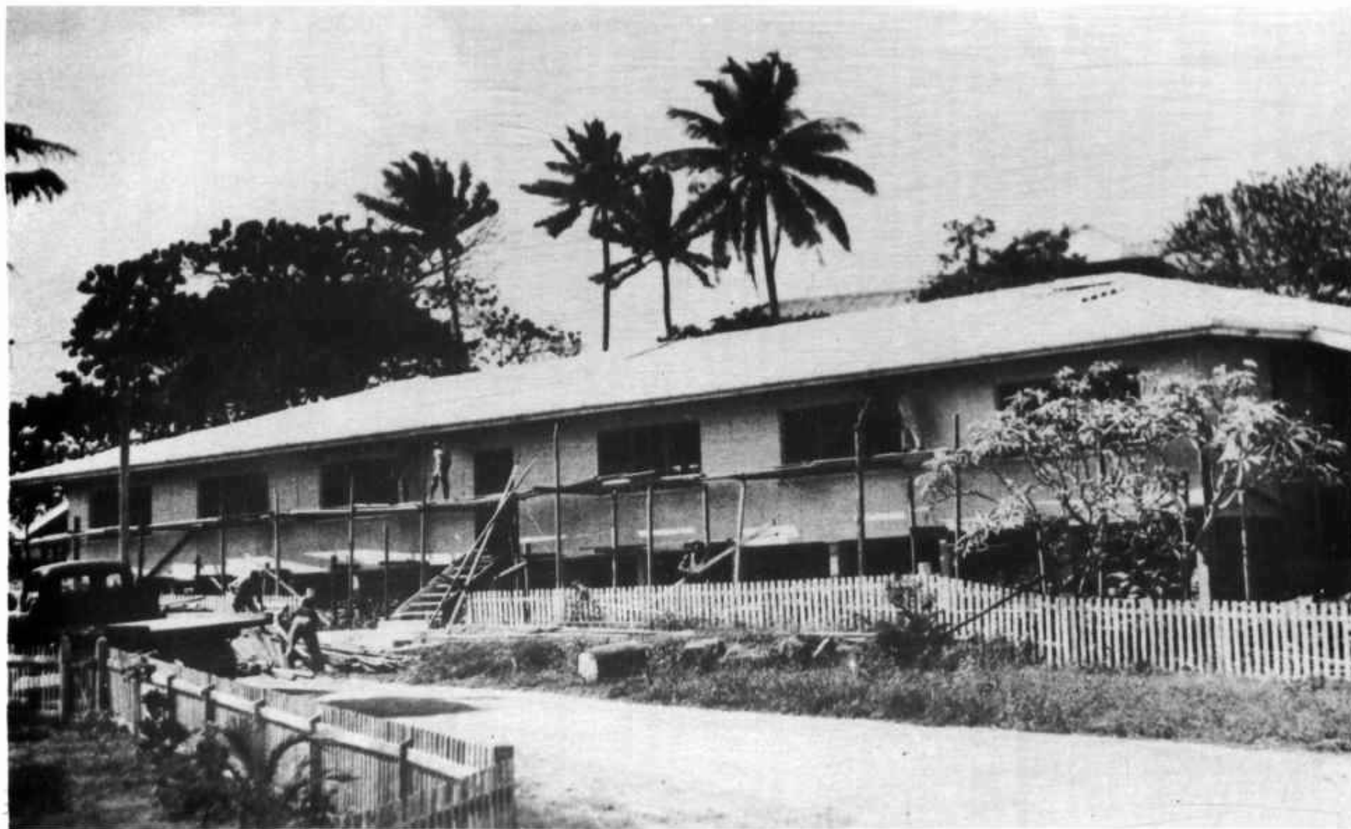
Erection of Coloured Nurses' Quarters and Domestic's Home, Thursday Island.
